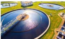
Industrial Water Treatment Plant
