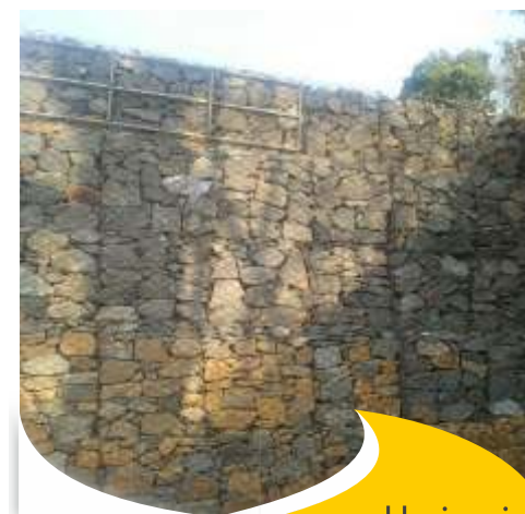
Lake Side Protection Gabion Wall
