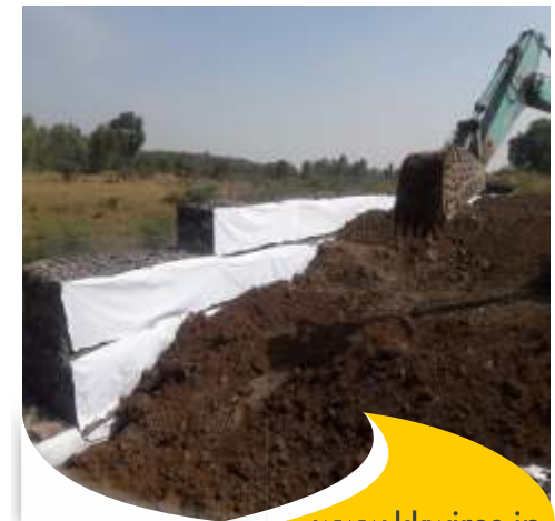
Warehouse Retaining Gabion Wall
