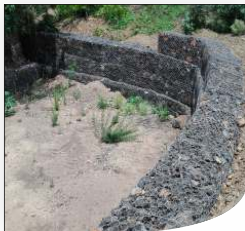
Dam Site Gabion Wall
