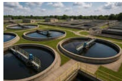
1000 KLD Industrial Sewage Treatment
