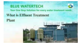
500 KLD MS Effluent Treatment Plant
