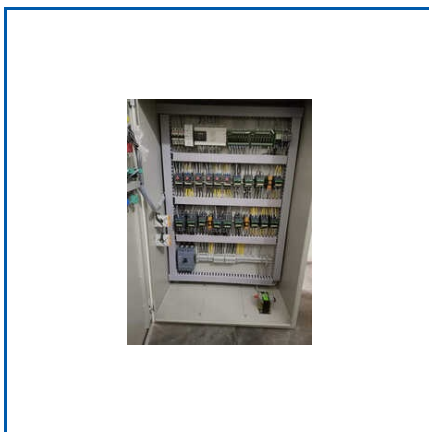
2000A FURNACE CONTROL PANEL
