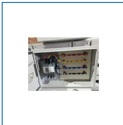
800A BUSBAR CONTROL PANEL
