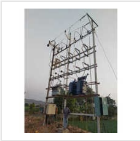
HT Electrical Work Services
