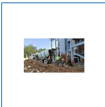
BUILDING CONSTRUCTION SERVICES
