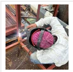
Civil Construction Work Services
