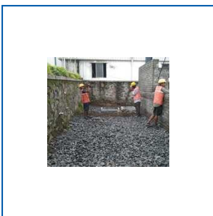
CONCRETE CHIPPING SERVICES
