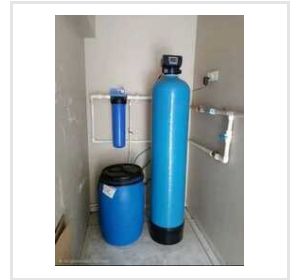
1000 Lph Water Softner RO Plant
