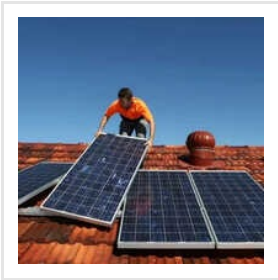
Solar Panels Installation Services
