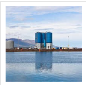
Sea Water Desalination Plant
