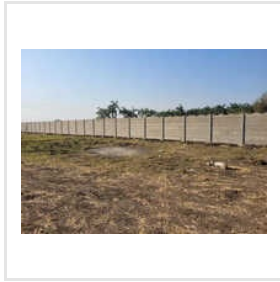
6ft Concrete Boundary Wall
