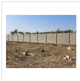
5ft Concrete Boundary Wall
