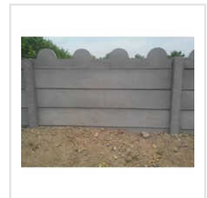
Compound Wall Construction Services
