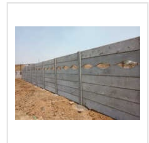
7ft Concrete Boundary Wall
