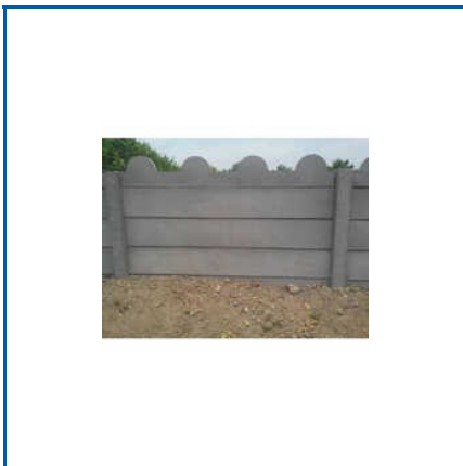
BOUNDARY WALLS CONSTRUCTION SERVICES
