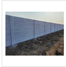
7ft Cement Compound Wall
