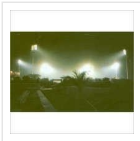
Stadium Lighting Poles
