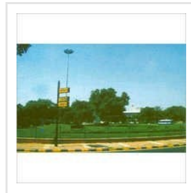
High Mast Lighting Poles
