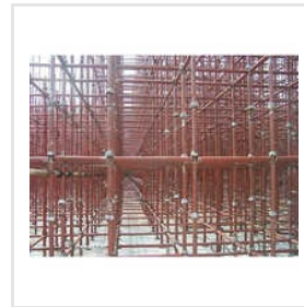
Construction Scaffolding System On
