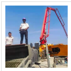
36 Meter Boom Pump On Rental Service
