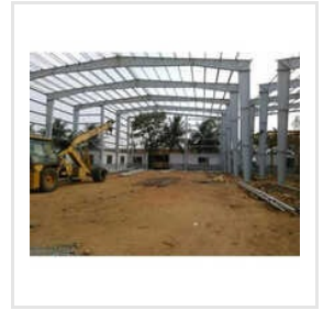
Structure And Truss Work
