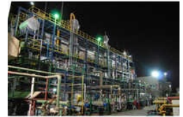
Fuel Ethanol Plant
