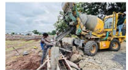
PEB RCC Construction Service
