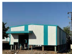
PEB Canopy Fabrication Services
