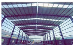
Industrial Roofing Services
