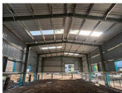
Skylight Installation Services
