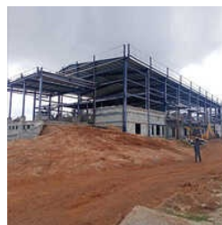
Multi Storey Steel Building Fabrication
