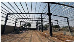
Steel Truss Fabrication Services
