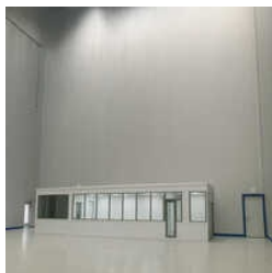
Shielding Room PD Labs
