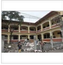
School Building Construction Services
