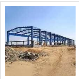
MS Prefabricated Building
