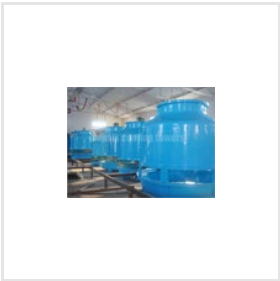
Round Shaped FRP Cooling Towers
