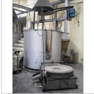
Industrial Lead Refining Plant
