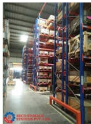
Drive In Racking System
