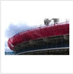
Construction Safety Net
