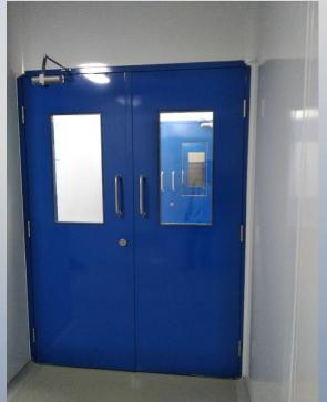
To maintain satirically correct air pressure in the room Doors are operated Manually by hand free operation and Automatic by hand sensor
