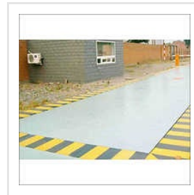
Concrete Pit Type Weighbridge
