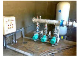
Hydro Pneumatic Pumping System
