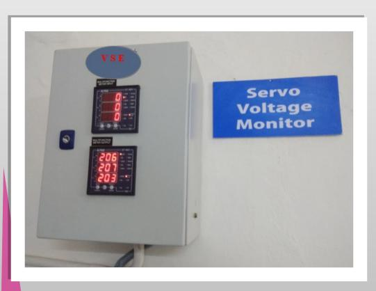
Servo Stabilizer Voltage Monitor with Three Phase Input and Output Voltage Monitoring with Scrolling and LED Indication with Hotter as an alarm
