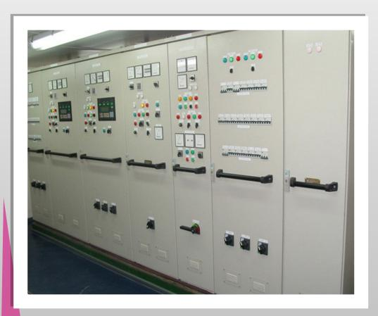
Synchronizing panels is used for synchronizing two or more DGs to share the total load of the system by matching all the parameter of the DG sets like voltage, frequency, speed, phase sequence and phase angle.
