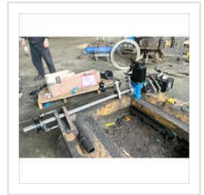
Line Boring Machine And Manual Welding
