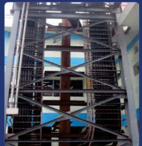
CABLE TRAY & LAYING
