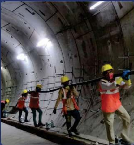
METRO UNDERGROUND CABLE LAYING
