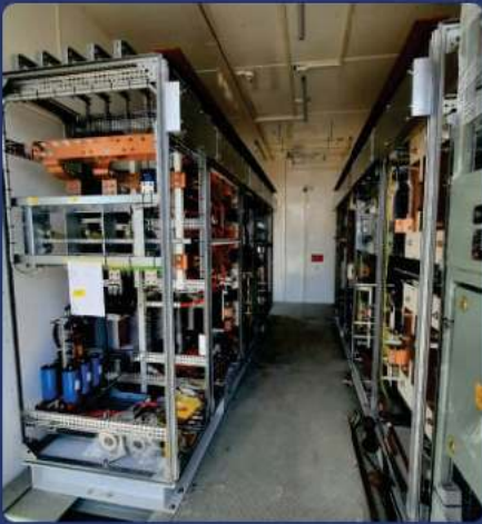
STATCOM PANEL INSTALLATION
