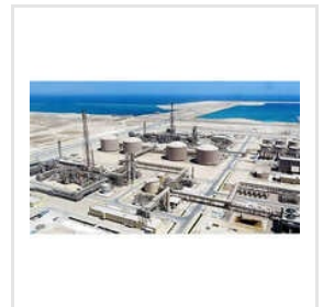
Sea Water Treatment Plant
