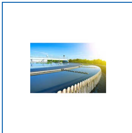
INDUSTRIAL STP PLANT
