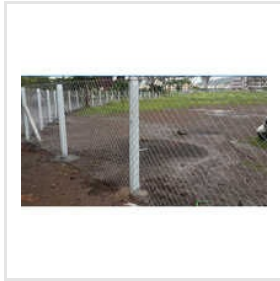
Cement Pole With Chain Link Fencing
