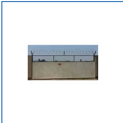
MS ANGLE WITH GI CHAIN LINK AND BARBED WIRE AND CONCERTINA COIL FENCING
