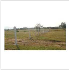
Cement Pole With Barbed Wire Fencing
