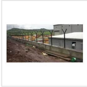
MS Angle Fixing Wall Fencing Job Works
