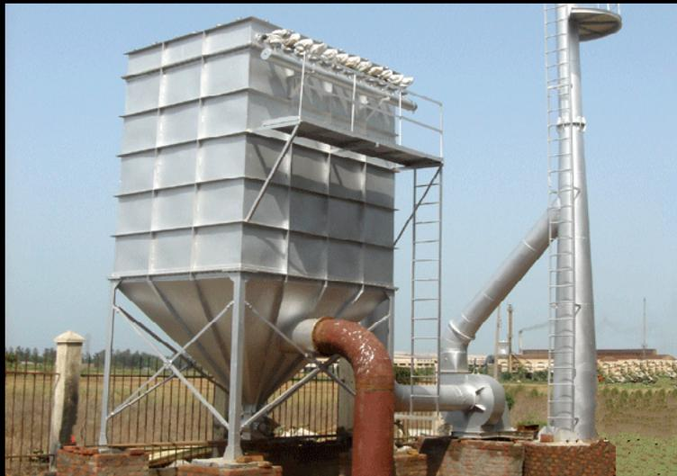
A **dust collector** is a system used to enhance the quality of air released from industrial and commercial processes by collecting **dust** and other impurities from air or gas. Designed to handle high-volume dust loads, a dust collector system consists of a blower, dust filter, a filter-cleaning system, and a dust receptacle or dust removal system. It is distinguished from **air cleaners**, which use disposable filters to remove dust.
