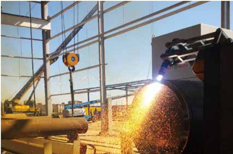
江苏前山管道制造车间内景 ▶ 车间面积：15000平方米 Outdoor scene, Jiangsu Qianshan pipe fabrication factory Factory area: 35000 square meters
