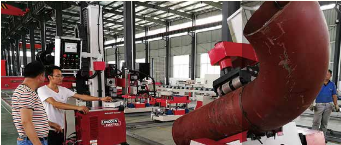
4、翻转式焊机窜动量测试 Swinging Pipe Welding Machine Displacement Measurement Test
