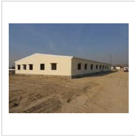
Prefabricated Office Structure
