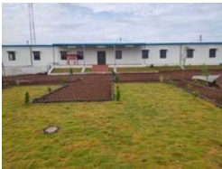
Prefabricated Staff Quarter
