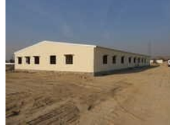
Prefabricated Office Structure
