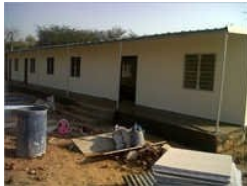
Portable Site Cabins
