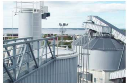
a structure for Application - Ash Handling Plant
