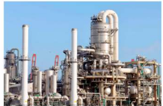
a structure for Application - Refineries
