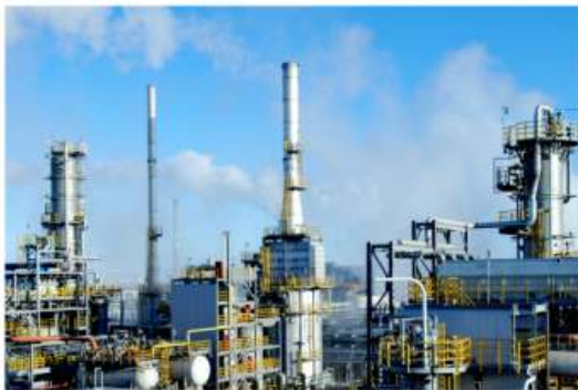
a structure for Application - Refineries
