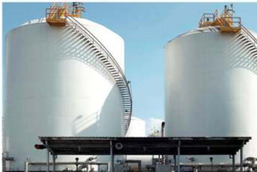
a structure for Application - Gas Storage
