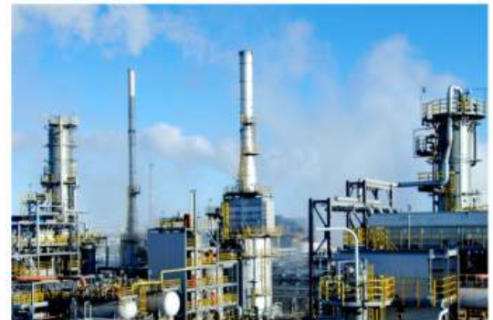
a structure for Application - Refineries
