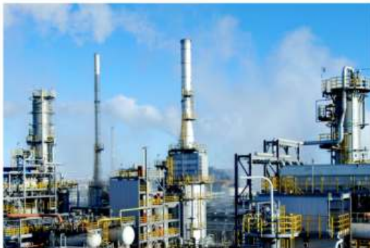
a structure for Application - Refineries
