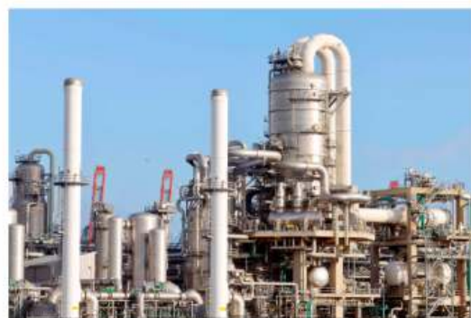
a structure for Application - Refineries
