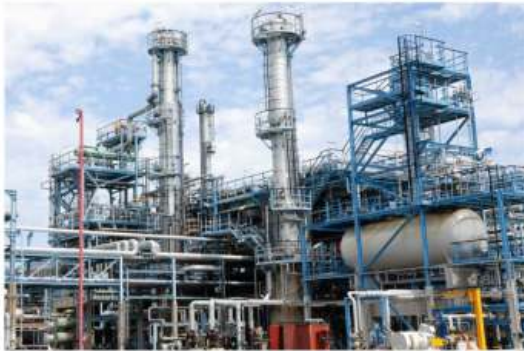
a structure for Application - Refineries
