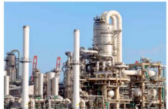
a structure for Application - Refineries
