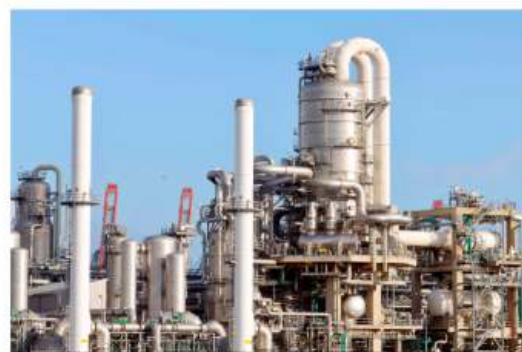
a structure for Application - Refineries
