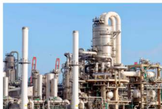
a structure for Application - Refineries
