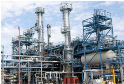
a structure for Application - Refineries
