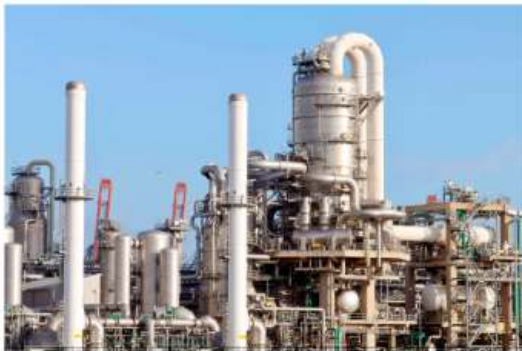
a structure for Application - Refineries
