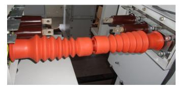
Sleeved busbars in coupled condition with insulating boot
