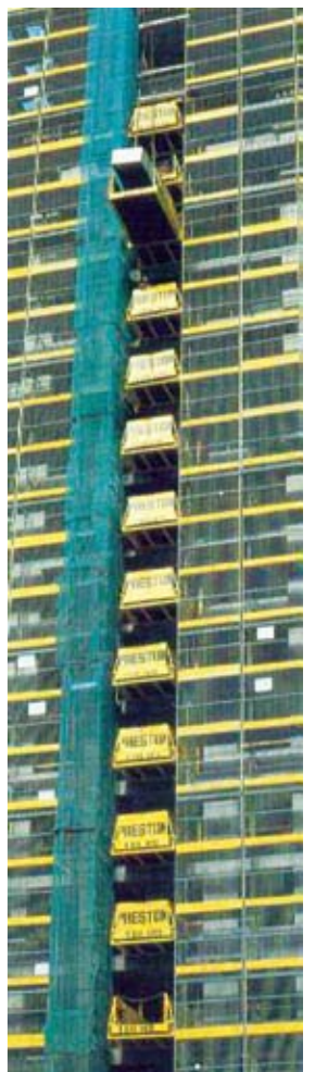
SUPERDECK used as overhead protection and loading platform
