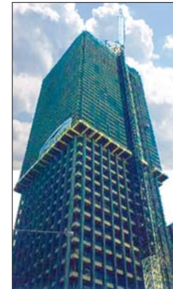
Overhead protection and scaffold support for demolition
