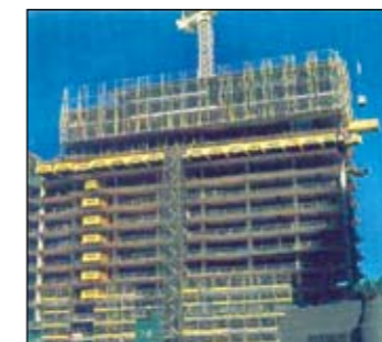
SUPERDECK used as overhead protection and loading platform
