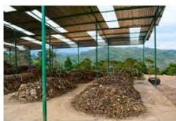
Solid Waste Treatment Composting Plant
