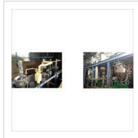
Lecithin Drying Plant
