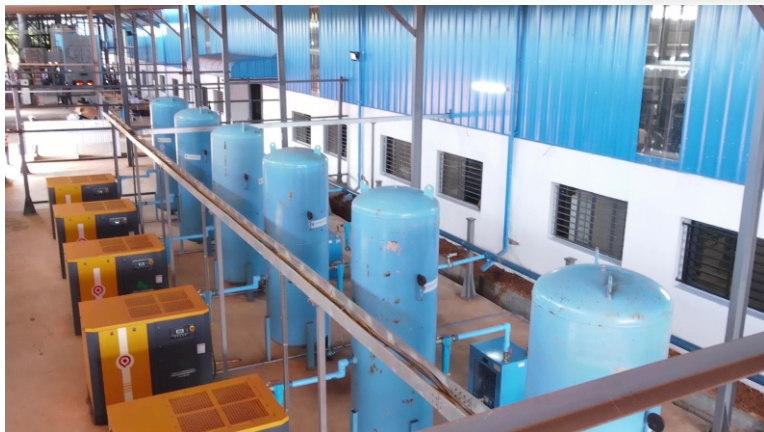
Cashew Peeling Section
