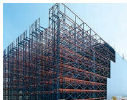
Rack Supported Warehouse
