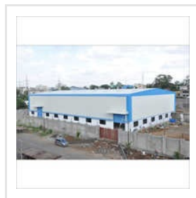
Mild Steel Industrial Shed
