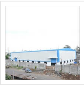
Prefabricated Factory Shed
