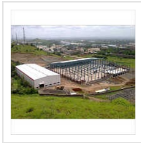
Galvanized Industrial Shed
