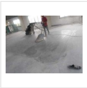
Concrete Floor Grinding
