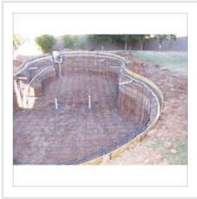
Swimming Pool Construction Services
