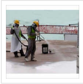
Commercial Floor Waterproofing
