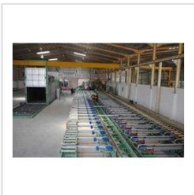
Aluminium Extrusion Plant Installation
