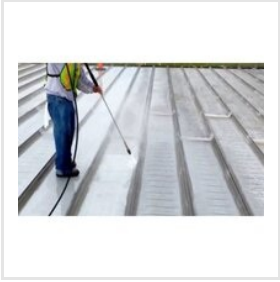
Cool Roof Coating
