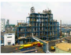
Stainless Steel Chemical Reactor
