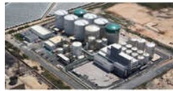
30kw Biodiesel Production Plant
