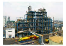
Chemical Process Equipment
