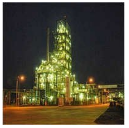
Plant Lighting Work
