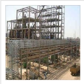
Electrical Contract Work
