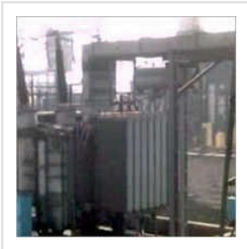
Transformer Erection Testing Services
