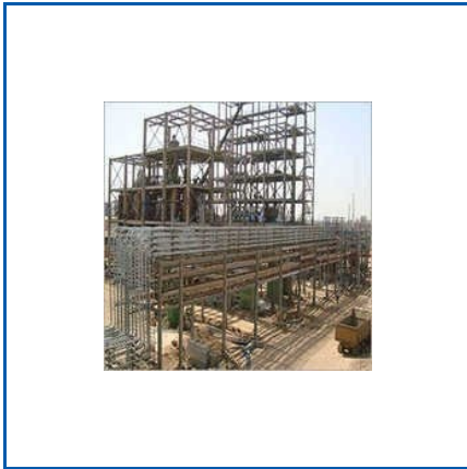
ELECTRICAL CONTRACT WORK
