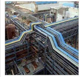
Electrical Installation Work
