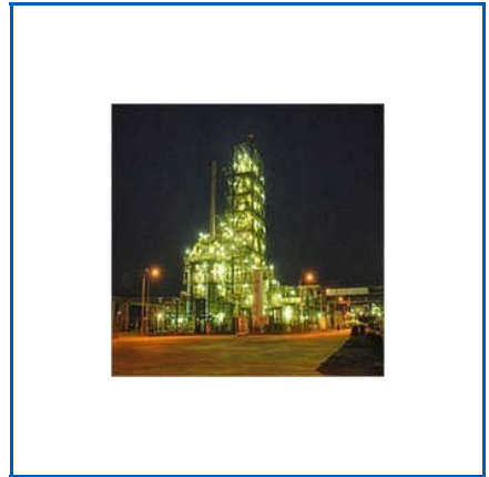
PLANT LIGHTING WORK
