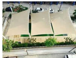
Swimming Pool Shed Structure
