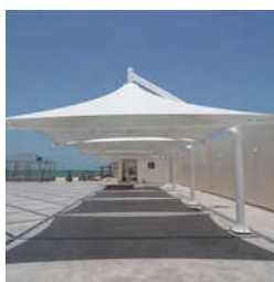
Gazebo Tensile Structure
