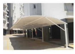
Commercial Car Park Canopy
