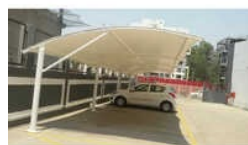
Car Parking Tensile Structure
