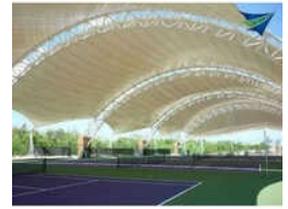
Auditorium Tensile Structure
