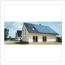
Solar Rooftop Systems
