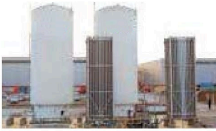
GAS to 6 MW Power Plant Installation
