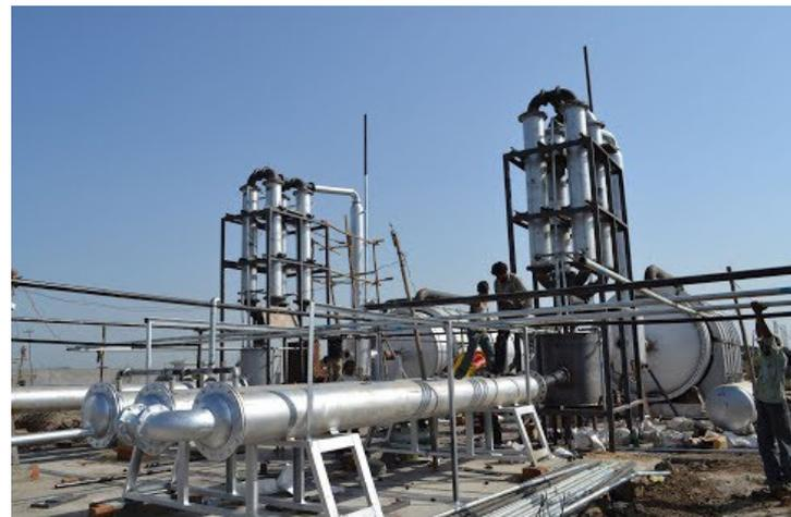
The pyrolysis plant is a machine converts mainly waste plastic/tyre to fuel oil. The raw material is waste plastic or waste tyre. The raw material will be heated in a reactor. When the oil gas goes into the condenser, the oil gas will be condensed into liquid oil/crude oil.
